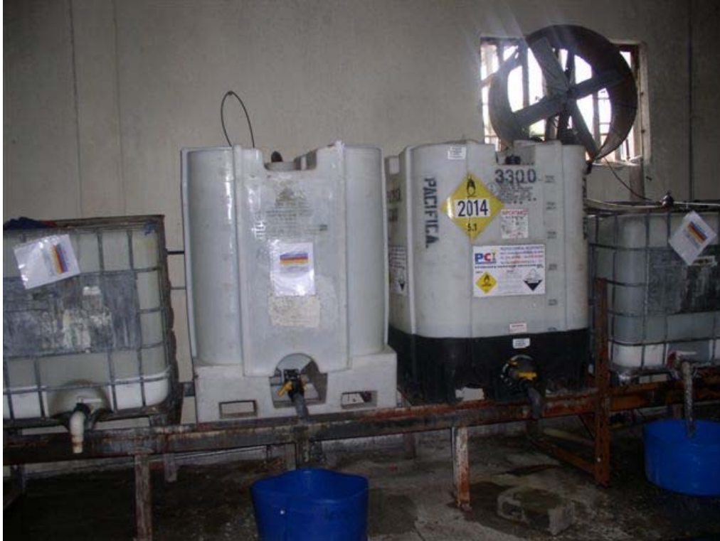
Exhibit 1. The chemical storage area where the incident occurred.
